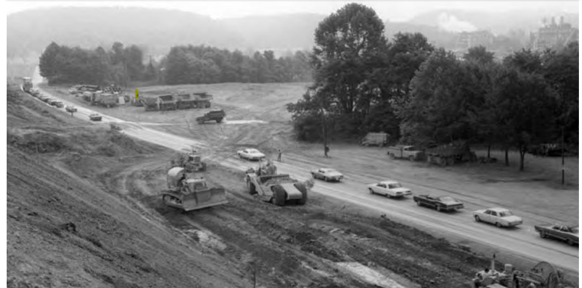
Route 460 Giles County Constructing 2 lane miles 1969
