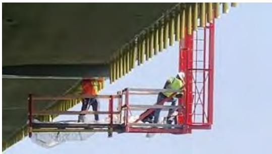
Installation of new scuppers
