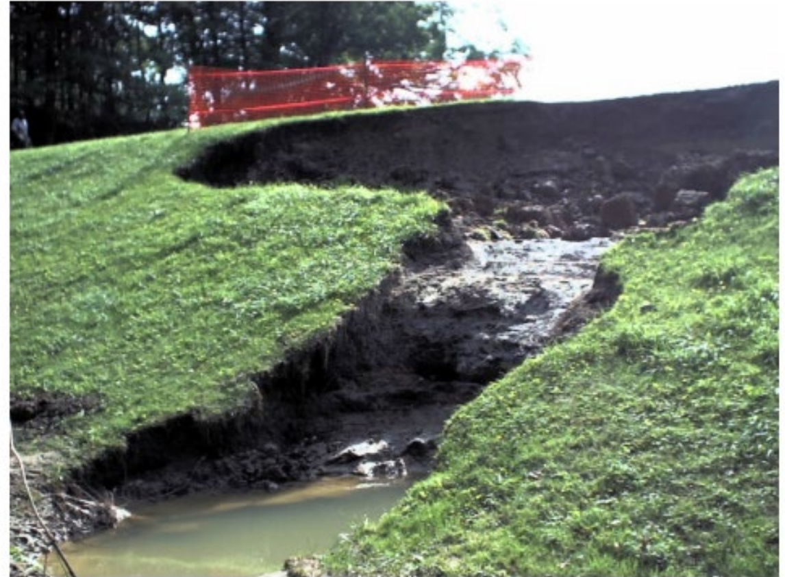
Figure 6-4.—Virginia Kendall Dam in Ohio after 3 hours of overtopping flow (Reclamation, 2003, courtesy of David Gillette).
