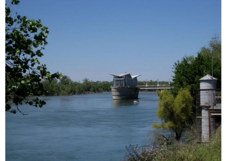
Example of a raw water intake
