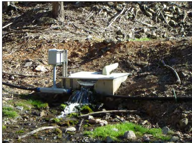
Seepage weir and collection box
