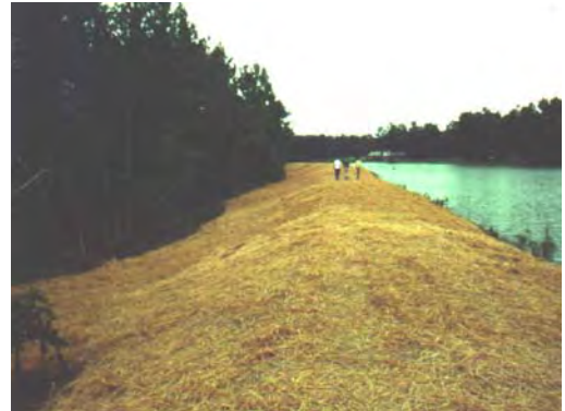
Figure 7. Completed remediation job after removing stumps, seeding, fertilizing & mulching.
