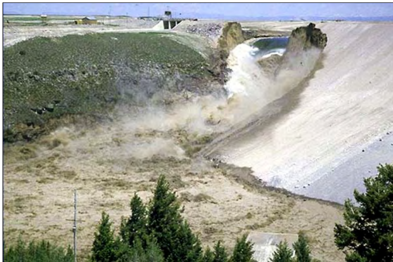
Failure of Teton Dam (Idaho) from seepage (1976)
