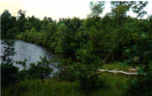
Figure 3. Example dam with inspection-hindering trees in Tennessee.
