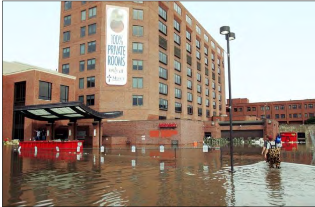
Flooding in Cedar Rapids, Iowa, including this hospital from overtopping of the spillway at Coralville Dam as a result of heavy rains (2008)
