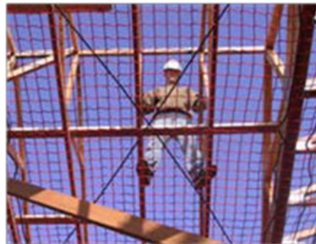
Figure 13. Safety net system.
