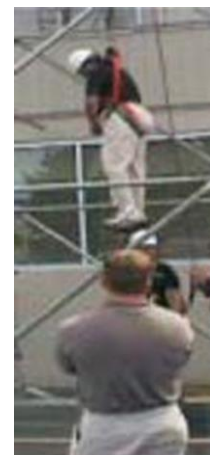
Figure 17. Worker suspended in harness prior to rescue.
