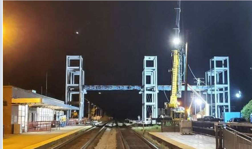
Pedestrian Bridge Construction at Quantico Station – August 2022.
