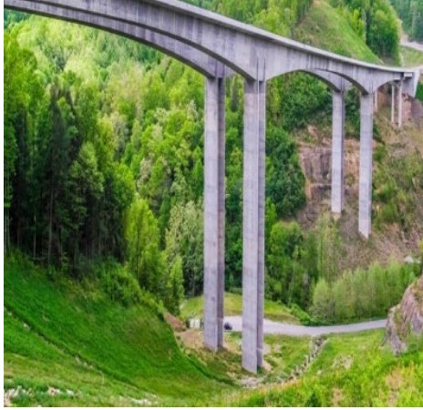
Grassy Creek Bridge (460 Connector)
