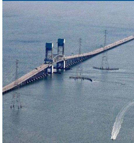
James River Bridge
