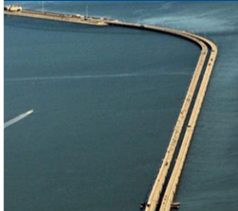
Monitor-Merrimac Memorial Bridge-Tunnel Approach Bridges
