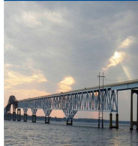
Robert O. Norris Bridge
