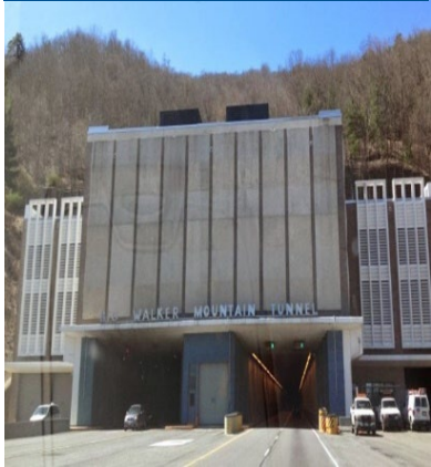
Big Walker Mountain Tunnel
