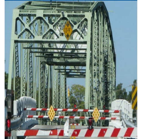
Gwynn's Island Bridge
