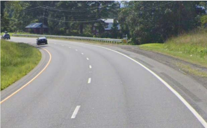
Paved Shoulder, Rumble Strip and Guardrail Example on Route 29
