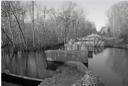
Carson Road (Rte 703) Bridge Replacement
