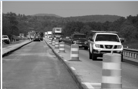
I-81 Pavement Project
