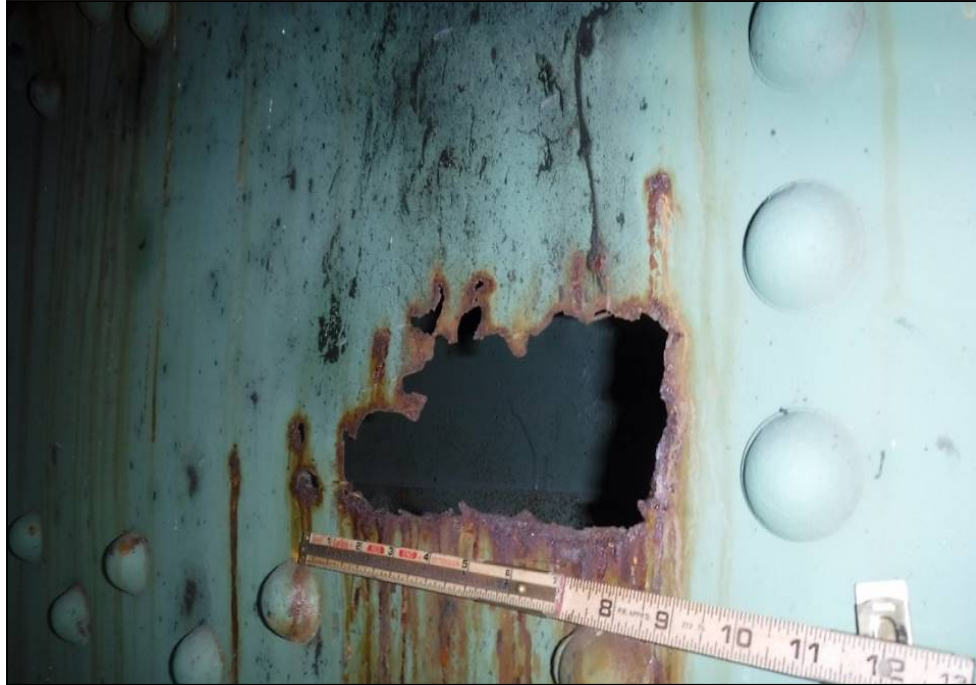
Cross Girder Repair
