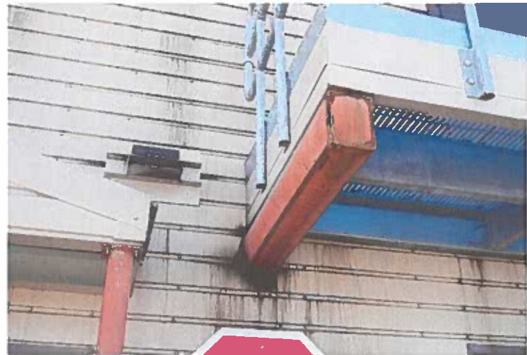
Winchester Re-Work 02-2023 026.JPG
