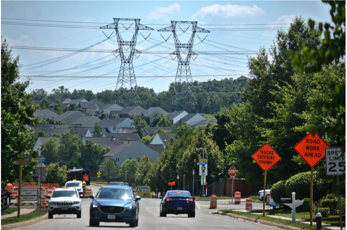
Power lines over homes in Kirkpatrick Farms, viewed from Supreme Drive in Aldie.
