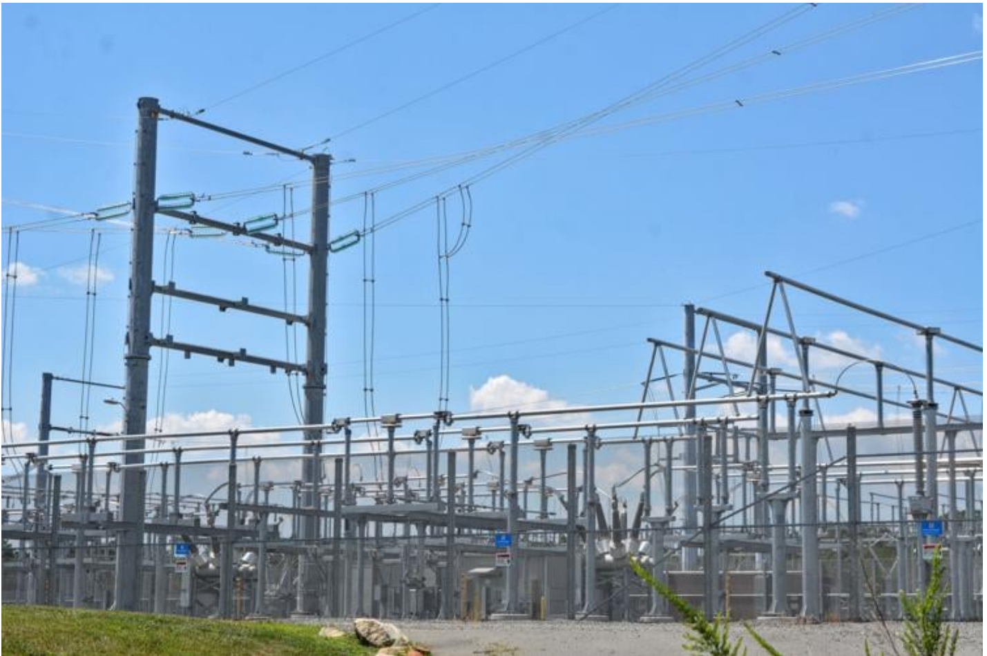
Power lines near the intersection of Old Ox Road and Loudoun County Parkway.
