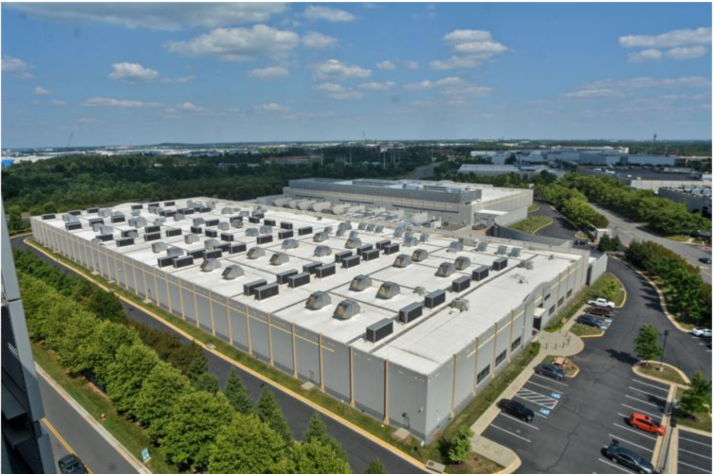
Data centers along Shellhorn Road, directly adjacent to Loudoun Station.
