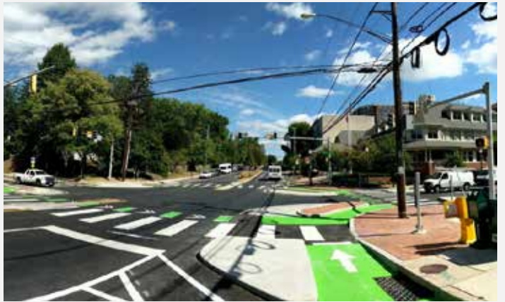
Figure 89: Protected Intersection in Montgomery County, MD. Photo by the Montgomery County Division of Transportation Engineering.
