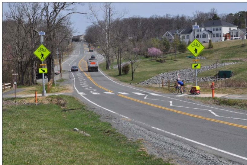
Figure 5. RRFBs and Signage at W&OD Trail Crossing
