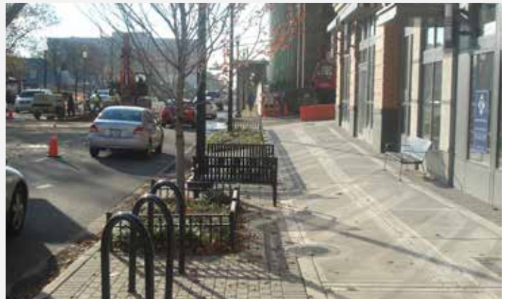
Figure 93: Bicycle Rack Placement in Arlington County. Obstructions like bicycle racks should be placed away from street corner areas. Bicycle racks should be placed in the amenity zone between the sidewalk and curb.
