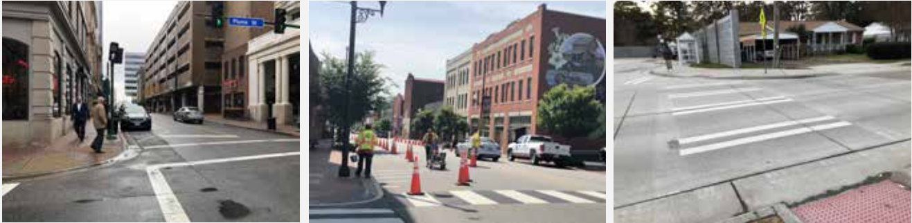
Figure 77: Example of Crosswalk Markings. From Left to Right: (1) Standard transverse lines in Norfolk, VA. (2) High-visibility longitudinal lines in Danville, VA. (3) High-visibility bar pairs in Norfolk, VA
