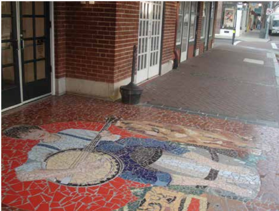
Figure 10: Decorative Sidewalk Paving in Roanoke. Decorative sidewalk paving not only enhances the pedestrian experience but can also connect visitors with local history.
