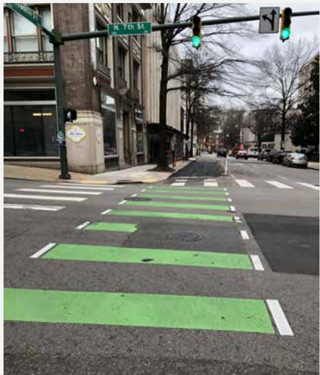
Figure 88: Green Dashed Pavement Markings for Bicycle Lanes Through Intersections . At the intersection of East Franklin Street and North 7th Street in Richmond, green paint supplements the white dashed lines indicating the continuation of the bicycle lane through the intersection. (Image Credit: EPR, P.C.)
