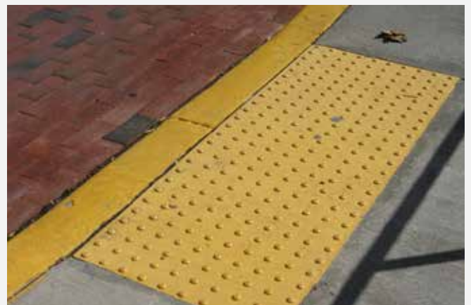
Figure 81: Detectable Warning Surface. Truncated domes are a surface treatment for curb ramps that alert pedestrians who are visually impaired that they are about to walk off a sidewalk into a roadway.
