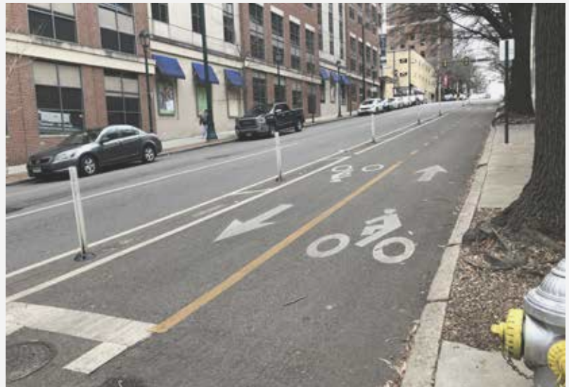
Figure 3: Franklin Street Two-Way Protected Bike Lane. The two-way bike lane on Franklin Street in downtown Richmond is one example of multimodal projects implemented in a variety of urban, suburban, and rural contexts since the Multimodal System Design Guidelines were first adopted in 2013. The City of Richmond has currently completed 32 miles of bike lanes, and more bike infrastructure projects have been designed and are in the pipeline. (Image Credit: EPR, P.C.)
