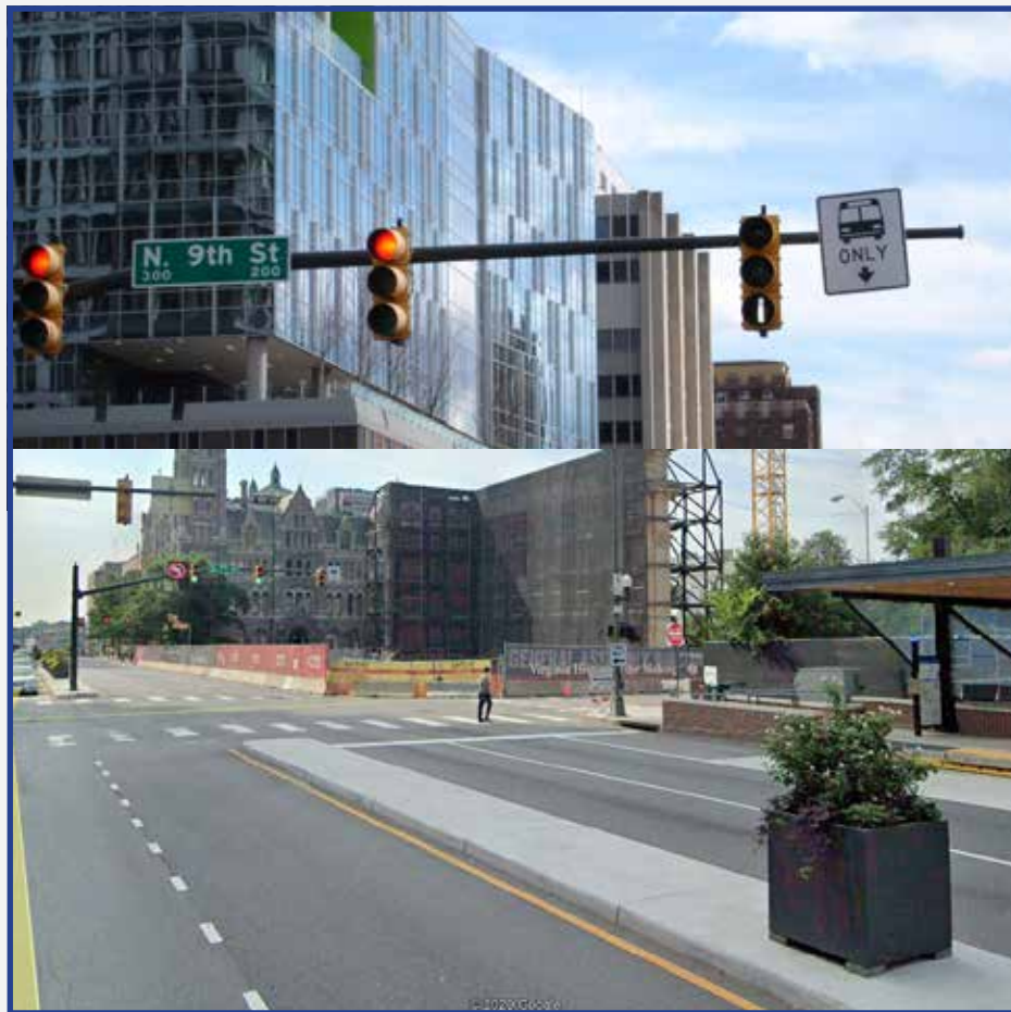
Figure 49: Broad Street Queue Jump at 9th Street, Richmond. Buses are given signal priority to get out in front of traffic. While the general traffic lanes have a red light, the vertical white bar indicates buses can proceed through the intersection. (Image Credits: VDOT (top), Google Earth (bottom))
