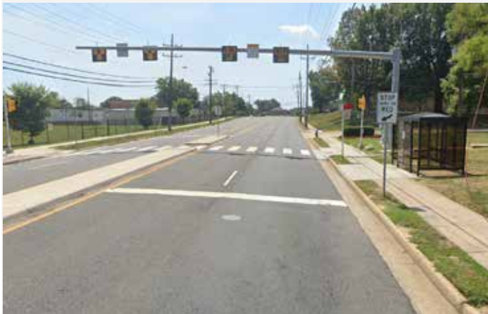
Figure 94: Pedestrian Hybrid Beacon in Fairfax, VA. (Image Source: Google Earth)
