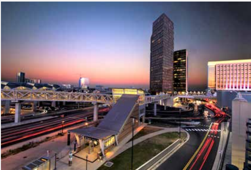
Figure 1: Tysons Corner Metrorail Station. The new Tysons Silver Line station and associated multimodal improvements at street level show the challenges and opportunities of retrofitting multimodal connectivity into existing contexts. (Image Credit: Wikimedia Commons).
