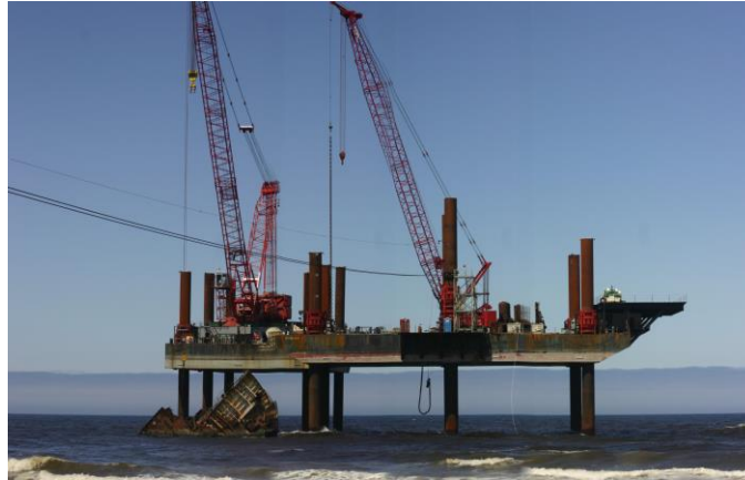
Barge with cranes held aloft on jacks.
