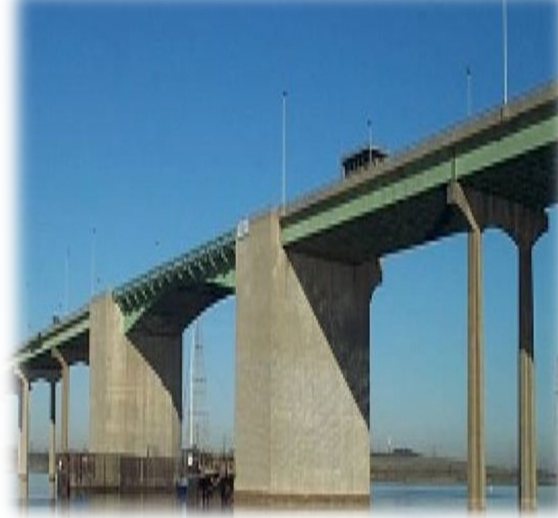
High Rise Bridge
