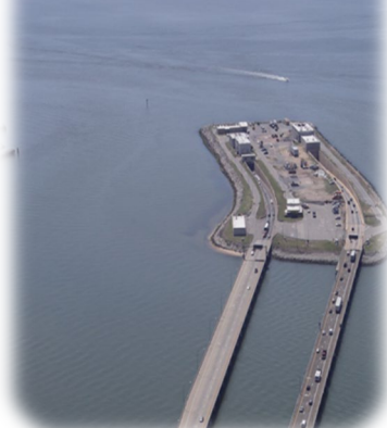
Hampton Roads Bridge-Tunnel
