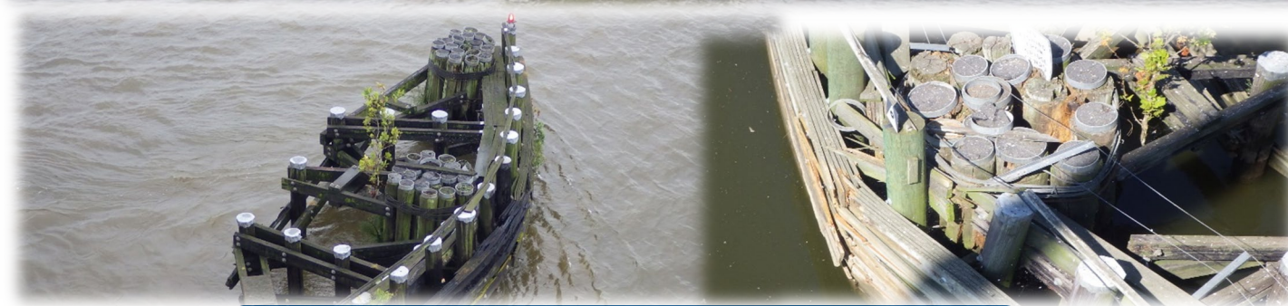
BEFORE: Old dolphins and fender (timber piles/wood)
