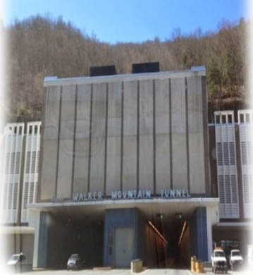
Big Walker Mountain Tunnel
