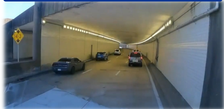
I-564 Runway Tunnel
