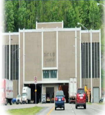
East River Mountain Tunnel
