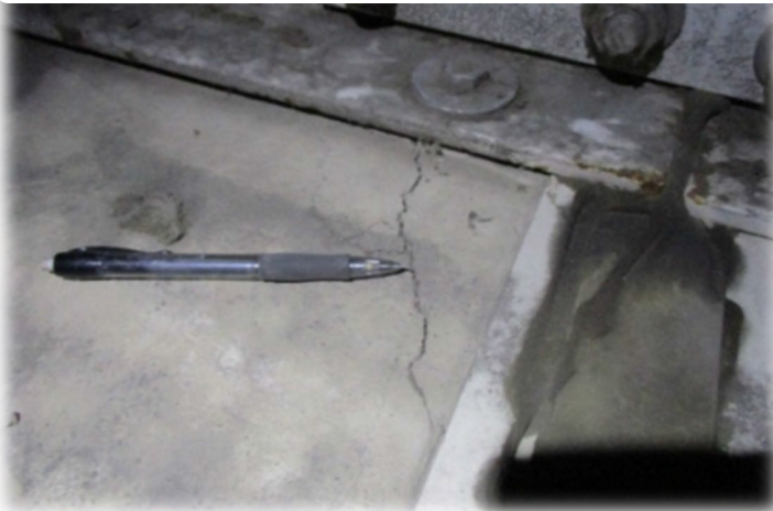
Cracked Ceiling Panel
