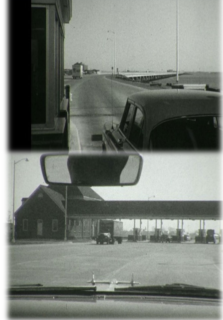
Hampton Roads Bridge-Tunnel
