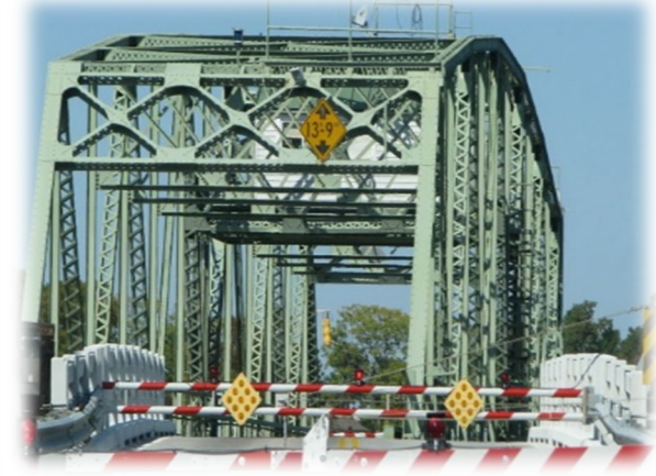
Gwynn's Island Bridge
