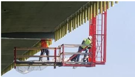
Installation of new scuppers
