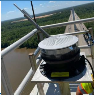
Installation of weather sensor
