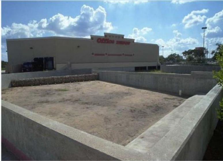
Figure P-FIL-06-2 Austin Surface Sand Filter
