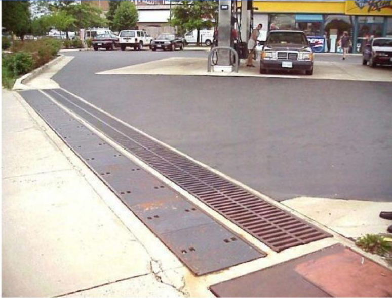
Figure P-FIL-06-3 Perimeter Sand Filter
