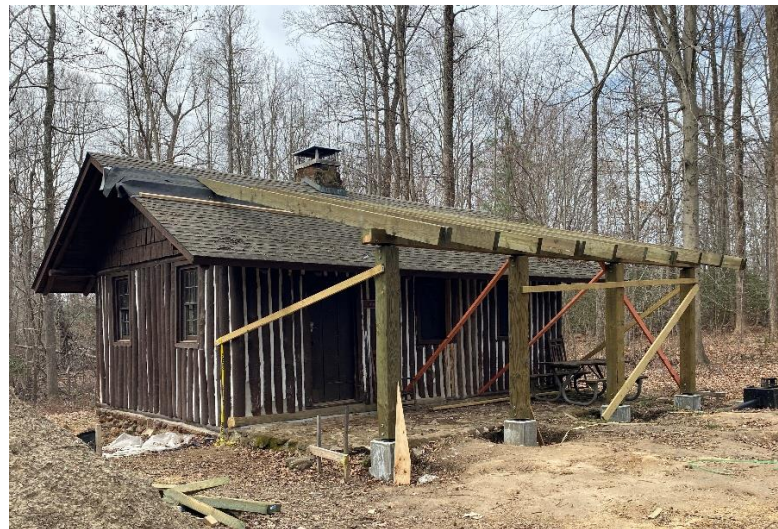
Figure 4: Westmoreland State Park: Cabin construction
