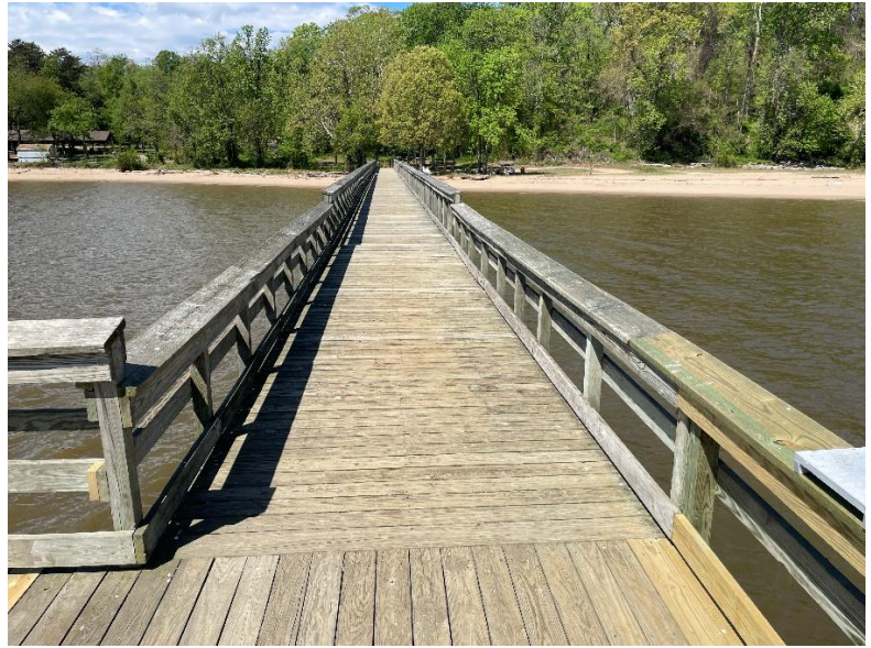
Figure 2: The pier at Leesylvania State Park
