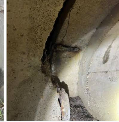
Joint separation/misalignment
