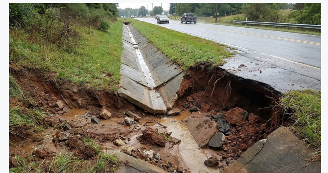
Undermining / Erosion
