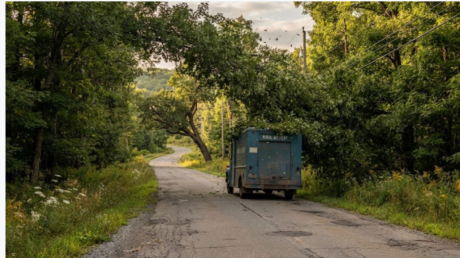
Vertical clearance over roadway
