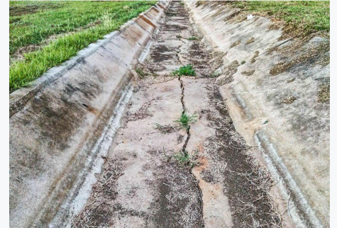
Cracking
