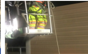
Sound Wall Repair
