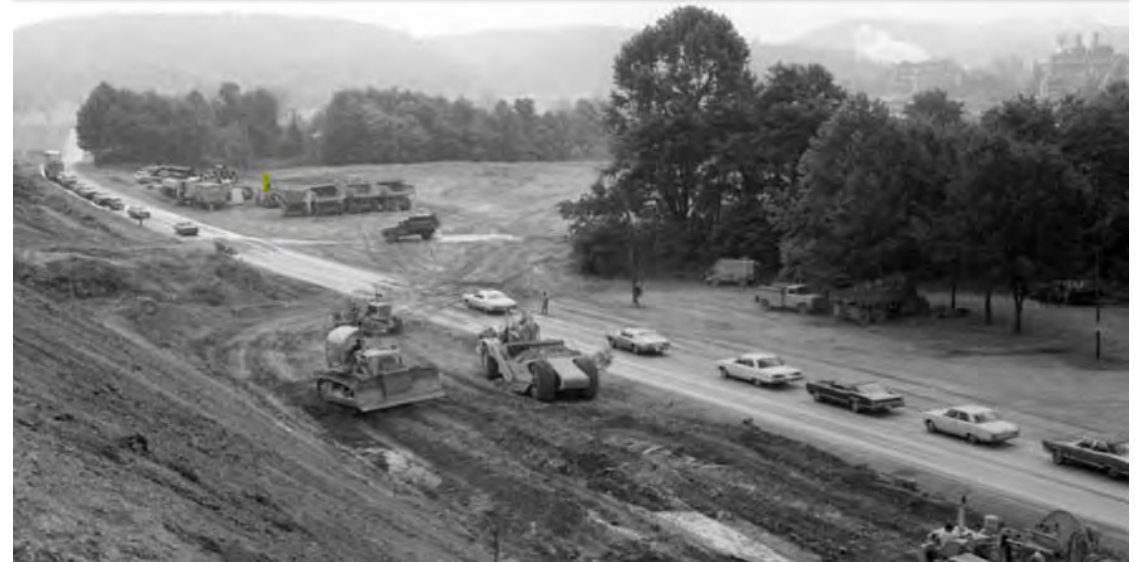
Route 460 Giles County Constructing 2 lane miles 1969
