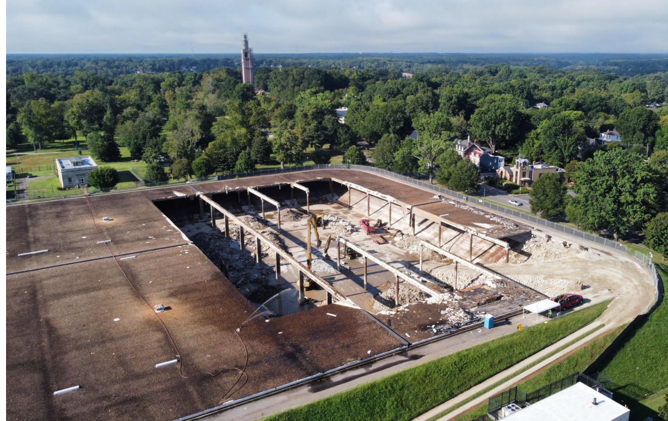
Byrd Park Reservoir, roof under construction
