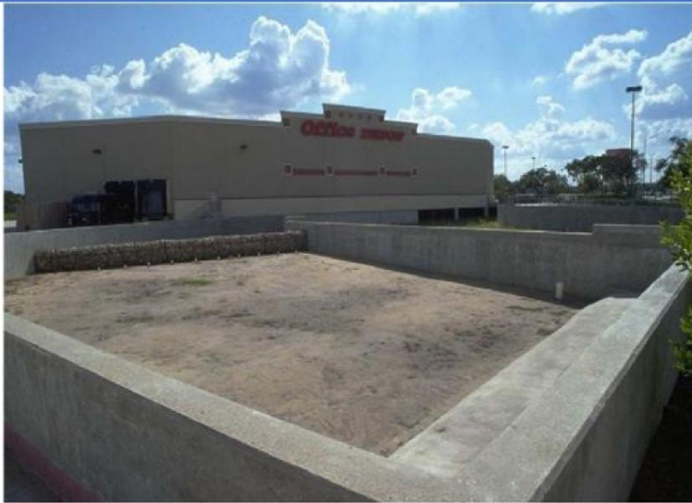
Figure P-FIL-06-2 Austin Surface Sand Filter
