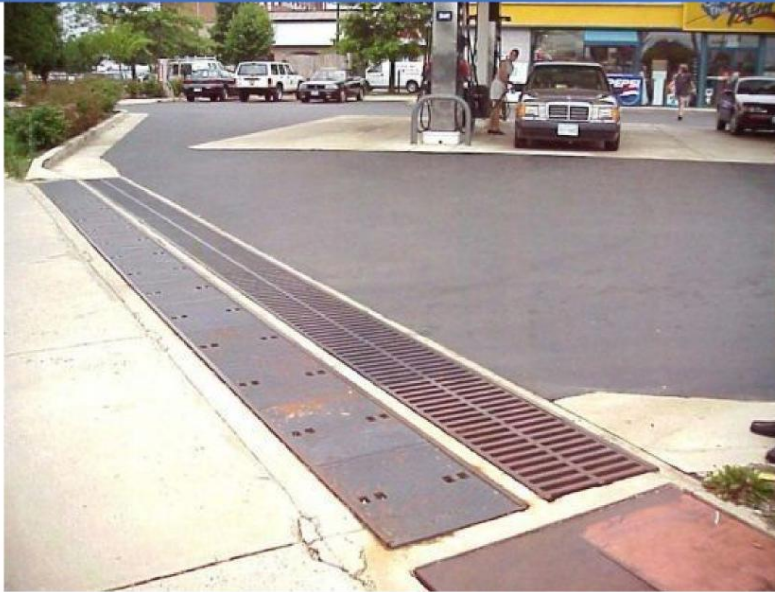
Figure P-FIL-06-3 Perimeter Sand Filter
