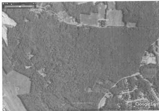
Figure 13. May 2006 aerial image of project area. Note the intact forest across much of the site.
