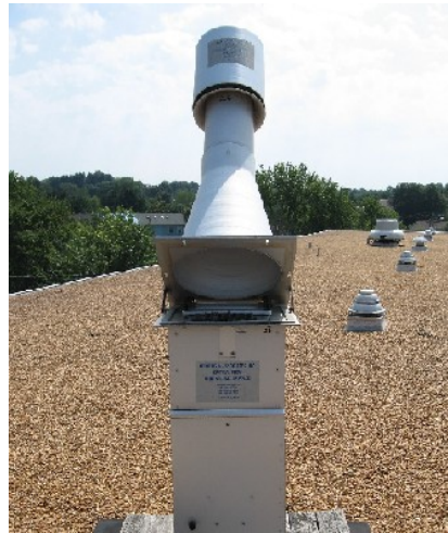
Inlet tilted on base front view
